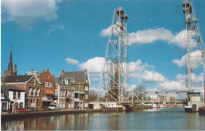
Vertical Lift Bridge over the river Gouwe in Boskoop
