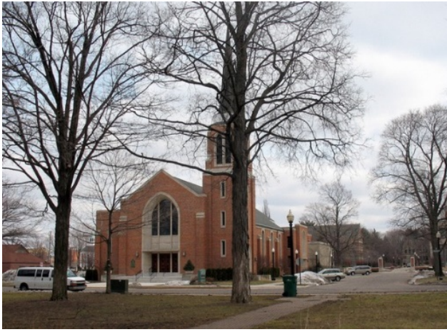
Central Avenue Christian Reformed Church
